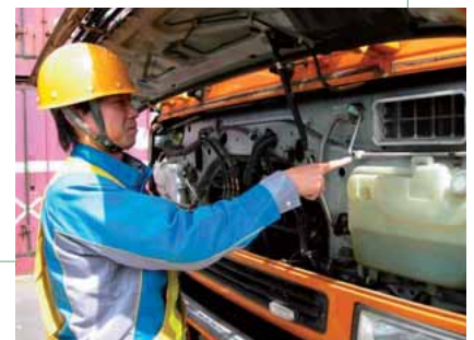
Air-conditioner gas status check using sight glass
