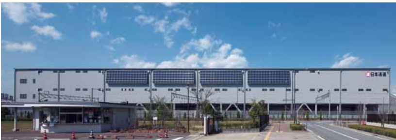
Tennoji Branch Logistics Centre
