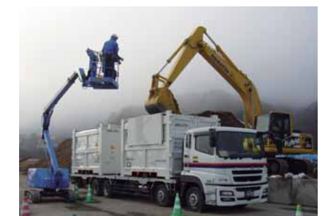
Loading up rubble in containers
