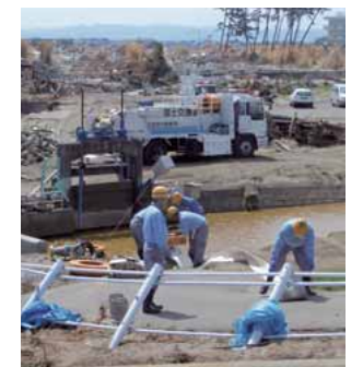
Draining water in the areas where floodgates had been damaged
