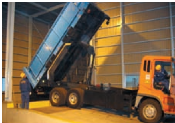
Sludge removal using open-top containers
