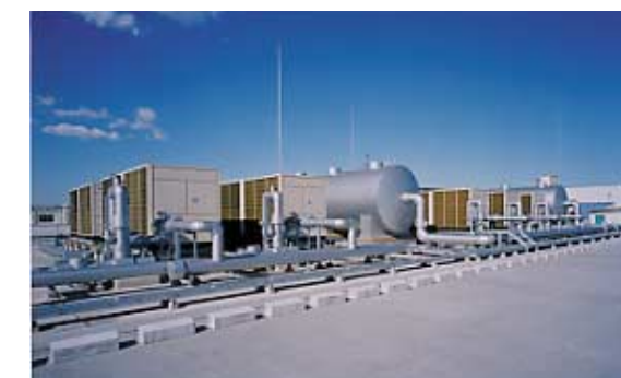
Low-temperature latent heat storage system
